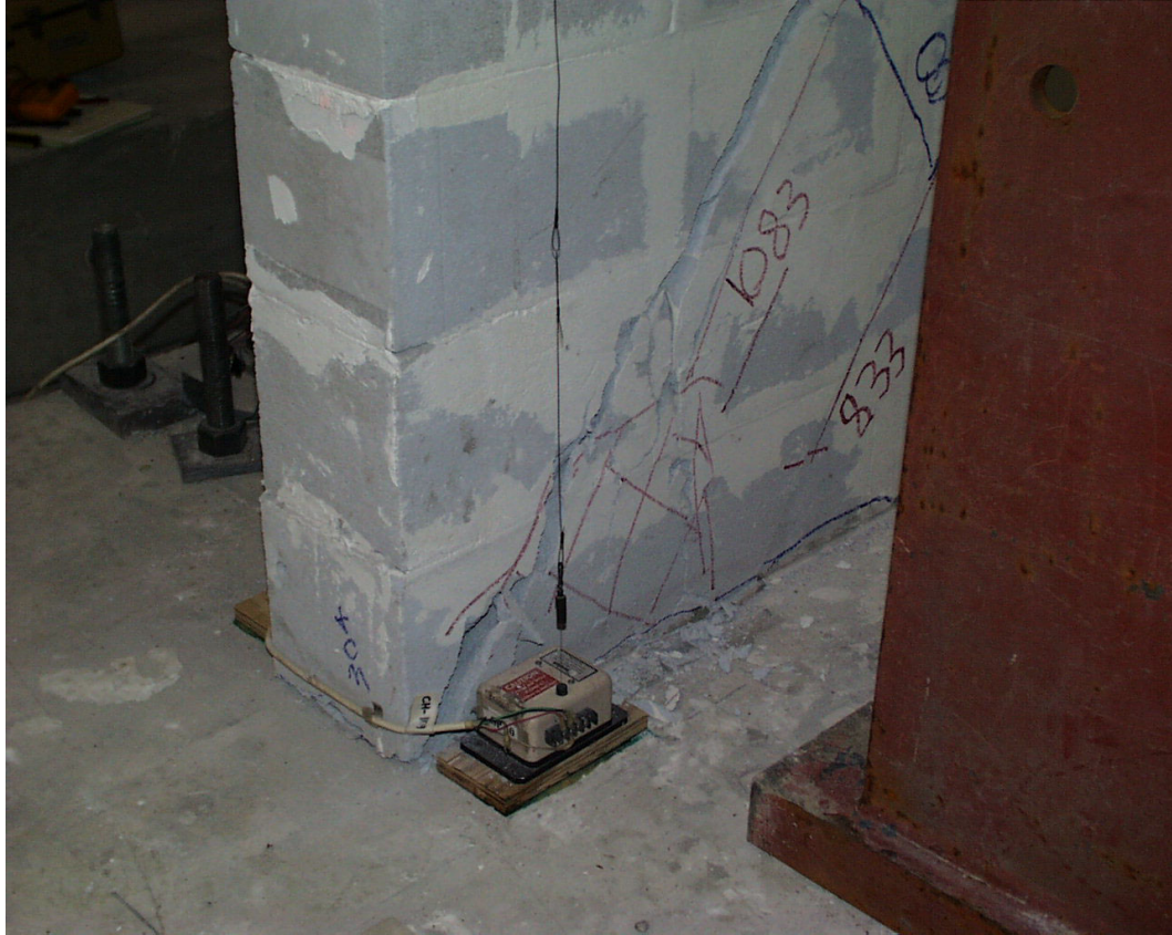
Figure 3.32: Toe crushing at the north end of Shear Wall Specimen 19
