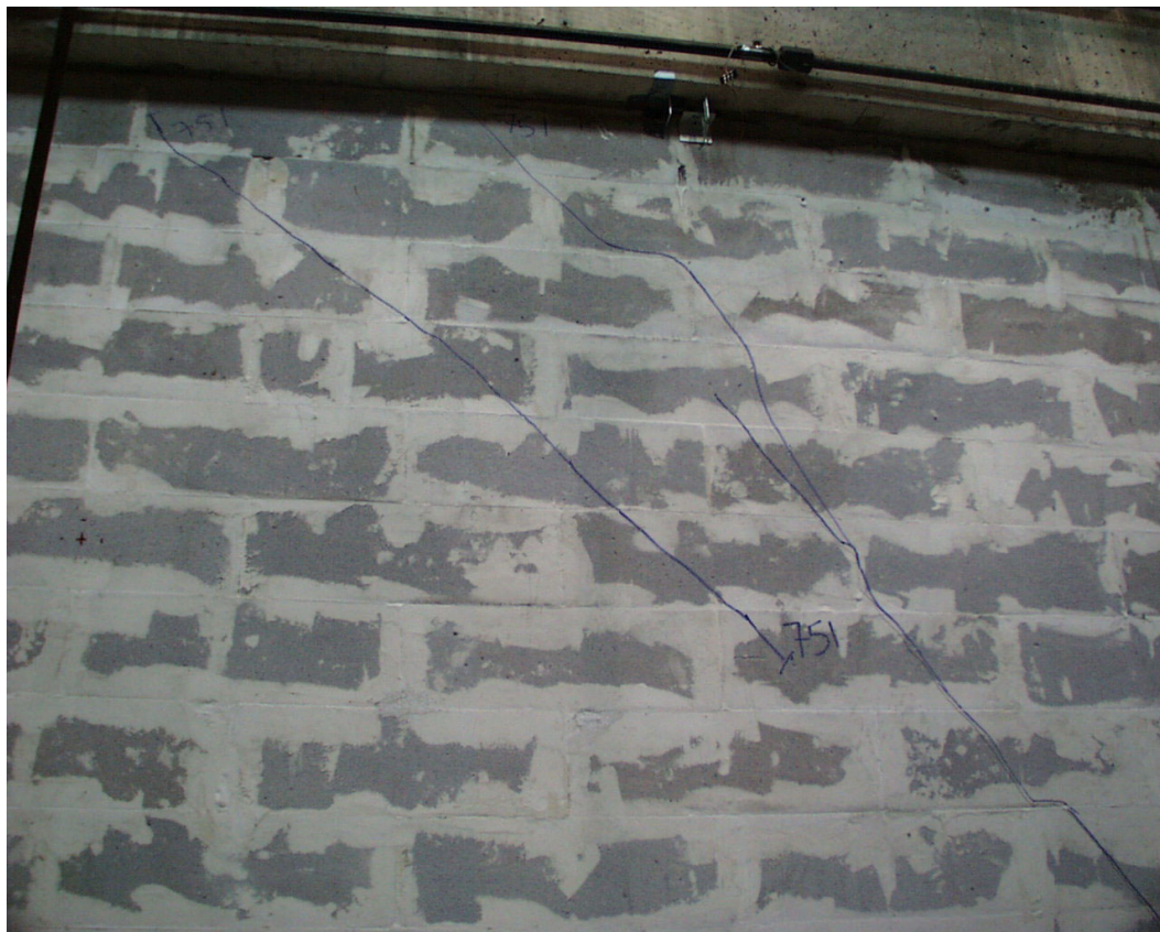
Figure 3.27: Web-shear cracking in Shear Wall Specimen 19
