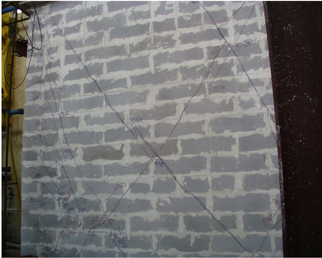
Figure 3.20: Web-shear cracks in Shear Wall Specimen 18
